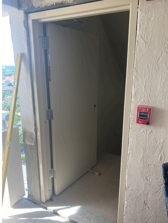
Picture 5: 7 th floor stairwell door in-progress installation
