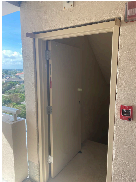
Picture 6: 6 th floor stairwell door in-progress installation
