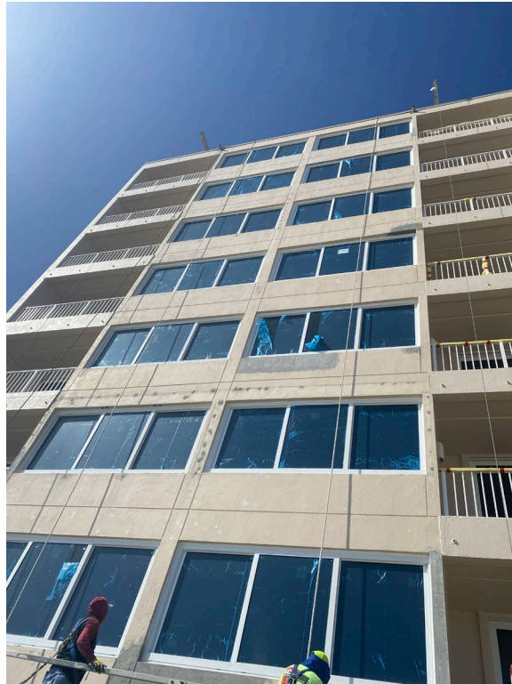
Picture 2: 10/11 window stack
