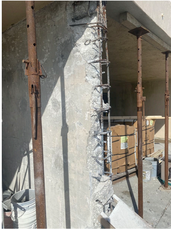
Picture 1: In-progress concrete repair
